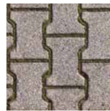
INTERNAL ROADS INTERLOCKING BLOCKS/ TREMIX CONCRETE ROAD
