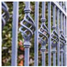
RAILING MS RAILING WITH ENAMEL PAINT FINISH
