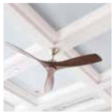
CEILING OIL BOUND DISTEMPER
